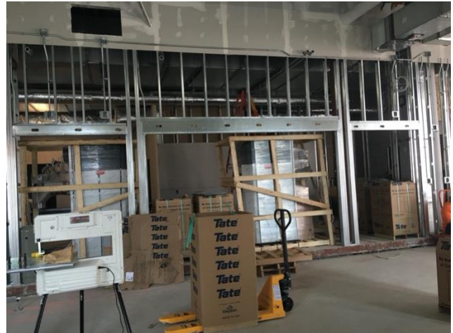
Figure 1 The Beacom Institute of Technology's Academic Server Room under construction
